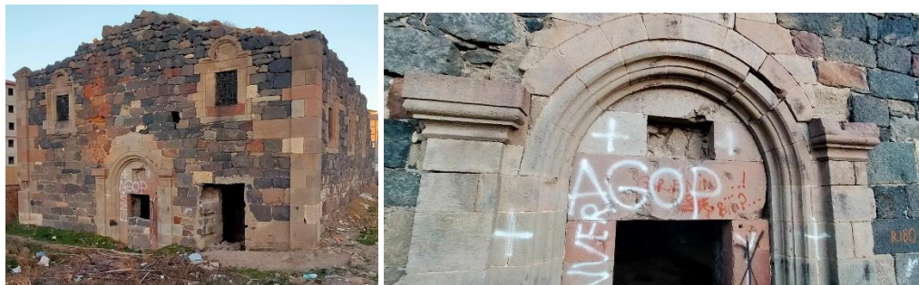
Photograph 3,4: Door General Photo (Personel Archieve 2021)
