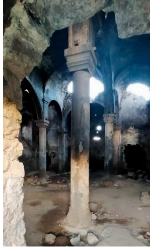
Photograph 5: Column (Personel Archieve 2021)
